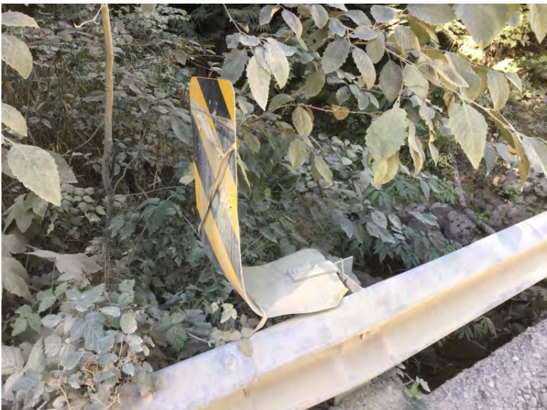
Delineator damage
