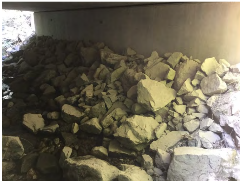
Left Bank Abutment when facing downstream
