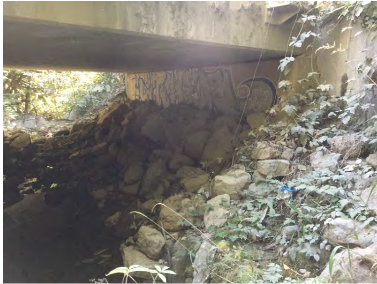
Right Bank Abutment when facing downstream
